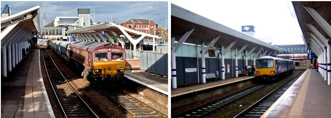
Figure 1.3 Freight and local passenger services at Rotherham Central
